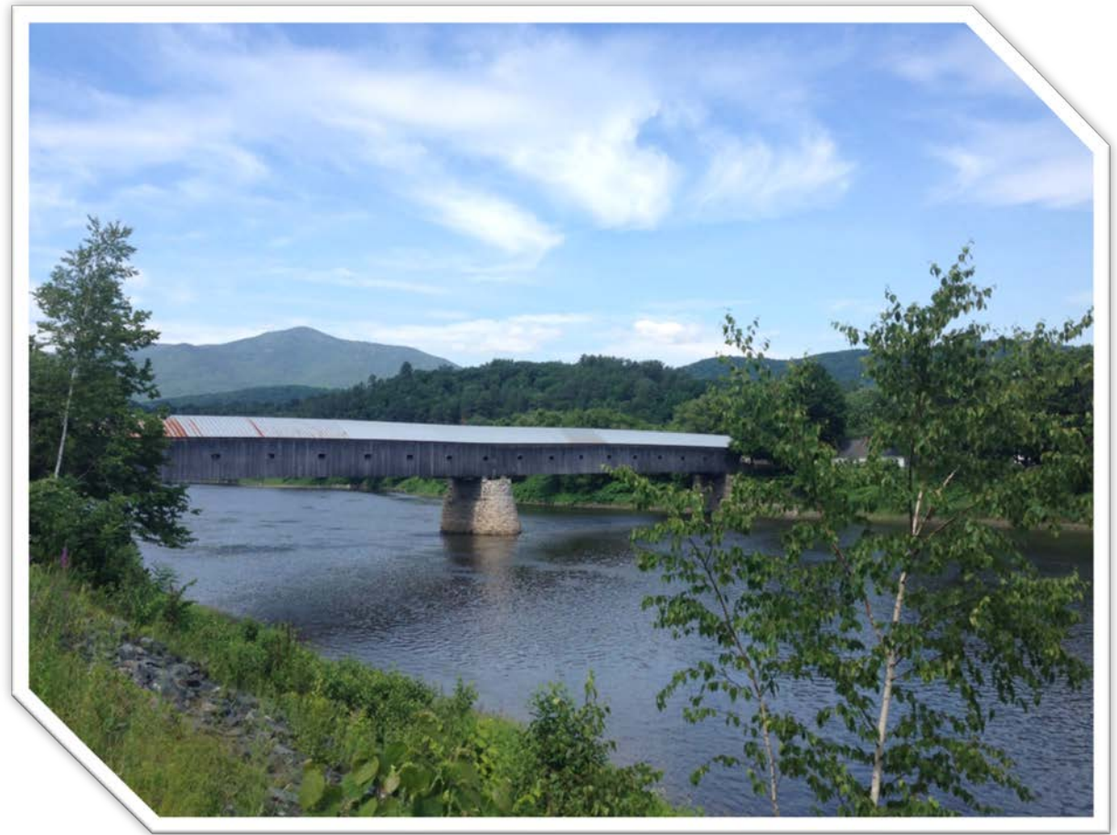
Cornish, NH Covered Bridge, Connecticut River
