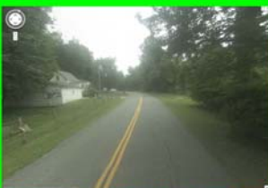
Pumping Station Road (Google Street View - 2009)
