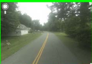
Pumping Station Road (Google Street View - 2009)
